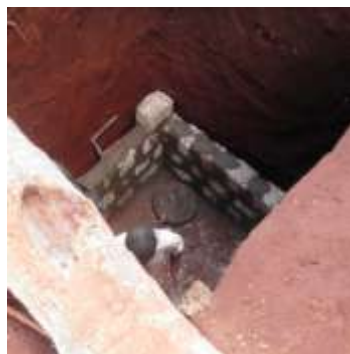
Digging the disposal pit
